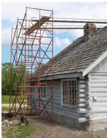
Rebuilding the chimney June 2014
